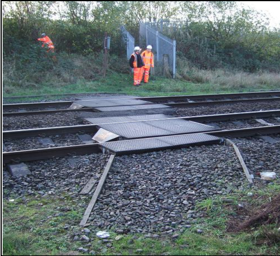
Figure 3: Moss Lane footpath level crossing looking south, November 2013
