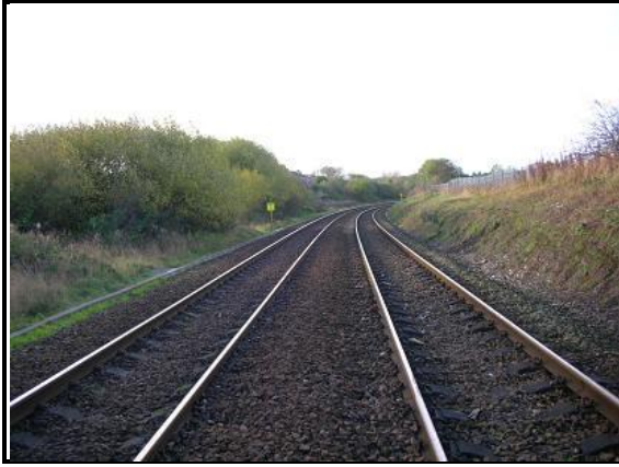
Figure 22: Down to Ashton Under Lyne approaching the crossing on the right side of the image. View from centre of Moss Lane level crossing looking west. November 2013
