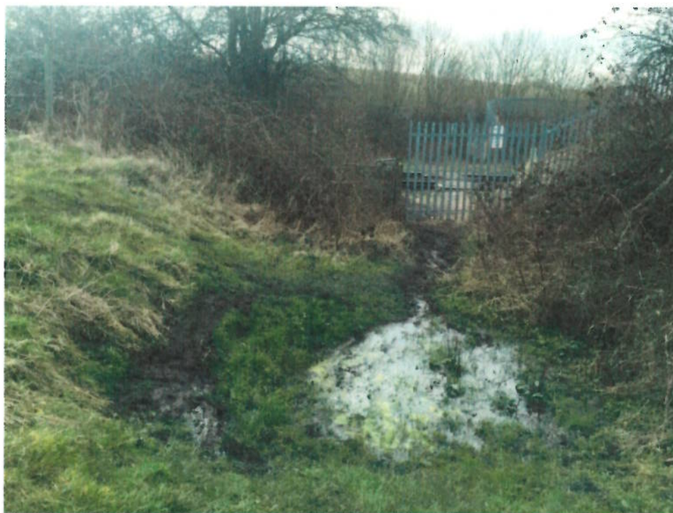
Flooding to north approach of crossing
