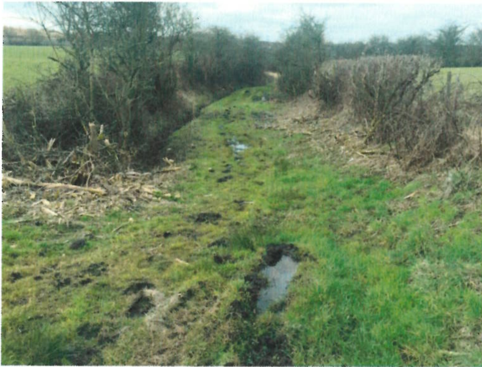
Uneven wet ground to north of footpath
