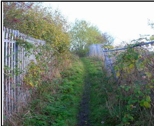
Figure 11: Un-surfaced footpath approaching Moss Lane footpath level crossing. Fence in poor condition on right of image. November 2013
