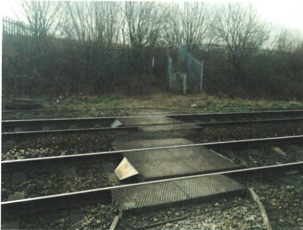
View on crossing from north looking south
