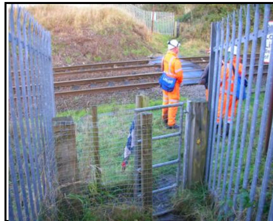
Figure 12: View of wicket gates at Moss Lane footpath level crossing. November 2013
