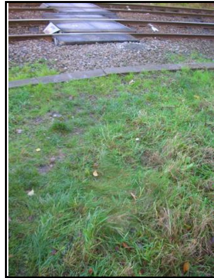
Figure 18: Ground condition approaching Moss Lane footpath crossing from the south. November 2013
