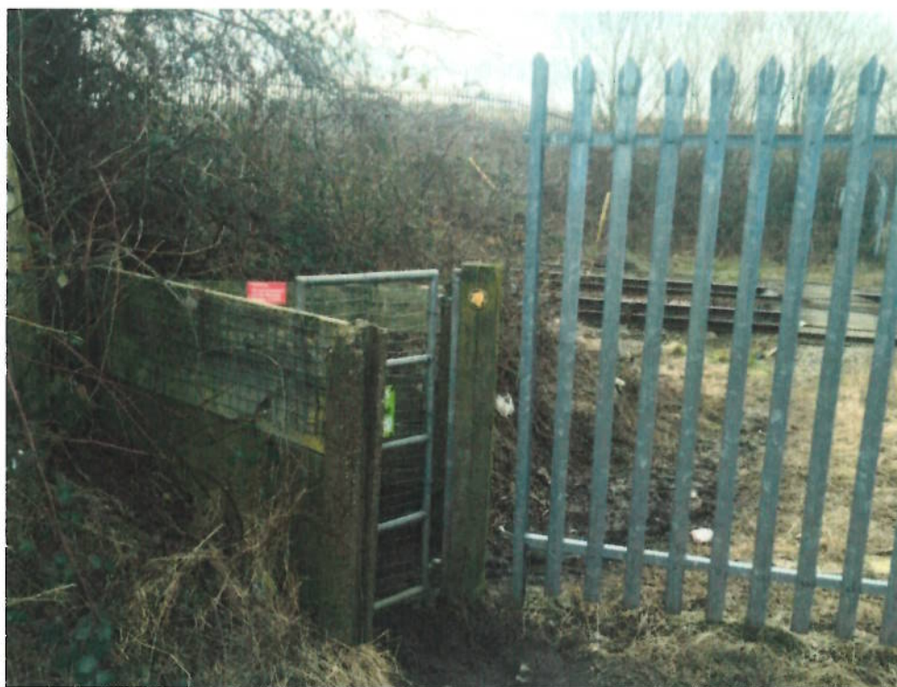
Gate / Fencing to north of crossing
