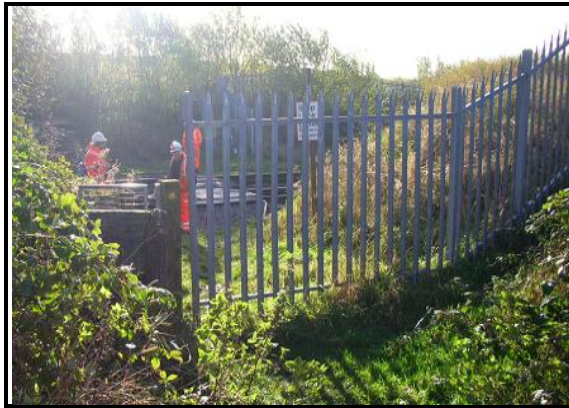
Figure 15: View of wicket gate on the left of the image and fixed palisade fencing on the right and centre of the image. November 2013
