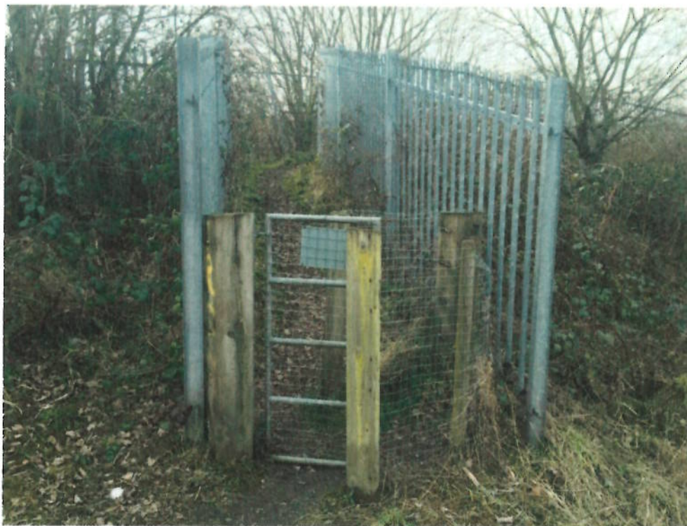
Fence and steep incline to south of crossing
